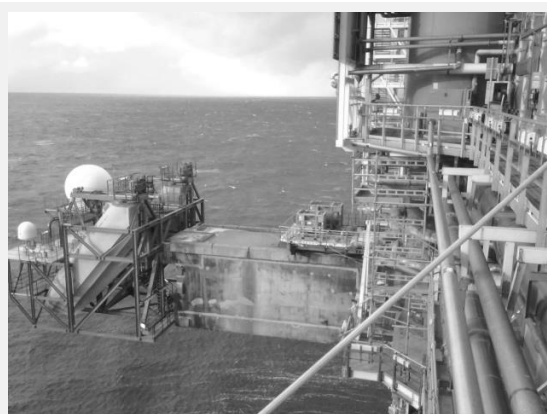
Figure 2. SWCTT location on the Heidrun platform.
